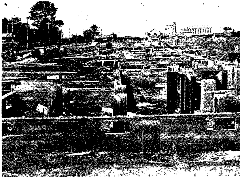
FOUNDATIONS LAID for the first block of houses on the big Government scheme on Oranga estate, Penrose.
